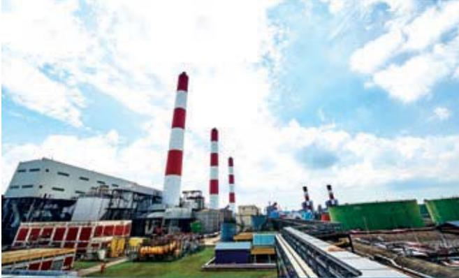
*The YTL PowerSeraya power plant in Singapore where almost 55% of the generating capacity has been converted from heavy fuel oil to natural gas*
