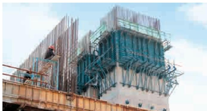
High early strength cement and concrete allow for faster formwork construction and removal
