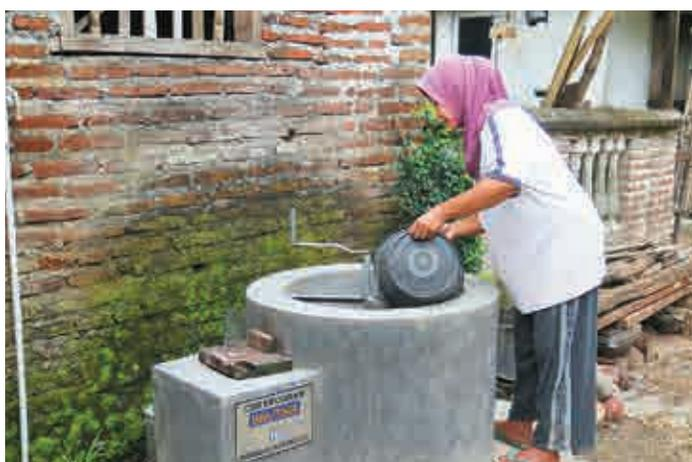
Cow dung being loaded into a biogas reactor unit
