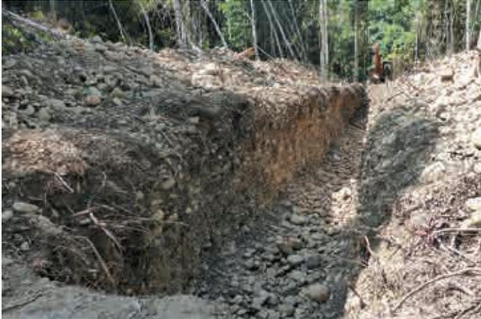
*Drainage excavated to ensure constant flow with sufficient gravity-feed energy to power the micro hydro at Kampung Iburu, Sabah*
