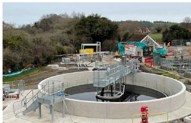
Storm overflow improvement project at Wessex Water
